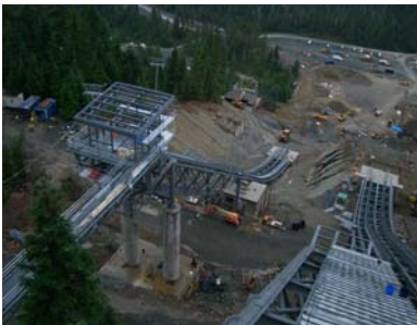
More than 700 tons of tubular steel was required for the fabrication of the ski jumps
