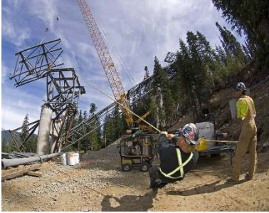
Field crew position a giant prefabricated truss into place.
