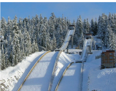
It took 3 months to completely erect the K-95 and K-125 jumps.
